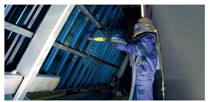
Fig. 3. Manual blasting of the exchange superstructure
